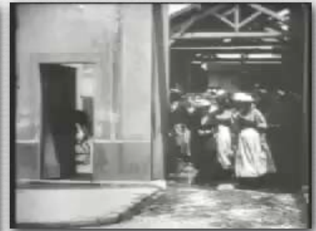
workers leaving the Lumière factory
